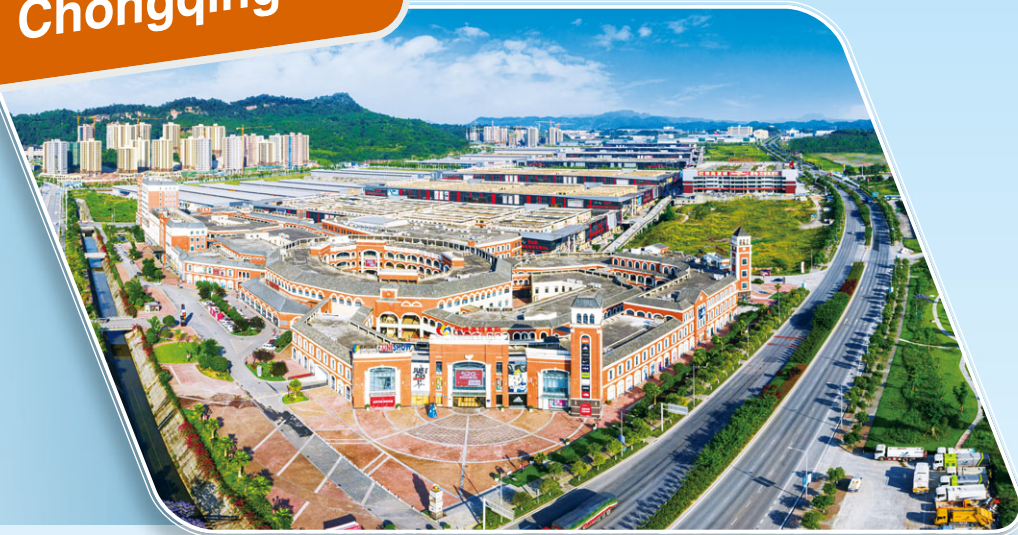
Huasheng Outlet and International Hardware Materials and Machinery Products Expo and Trade Centre in CSC Chongqing
